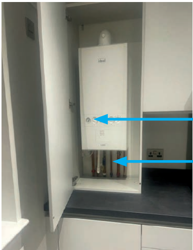
Pressure gauge Pressure top up valves situated below boiler
